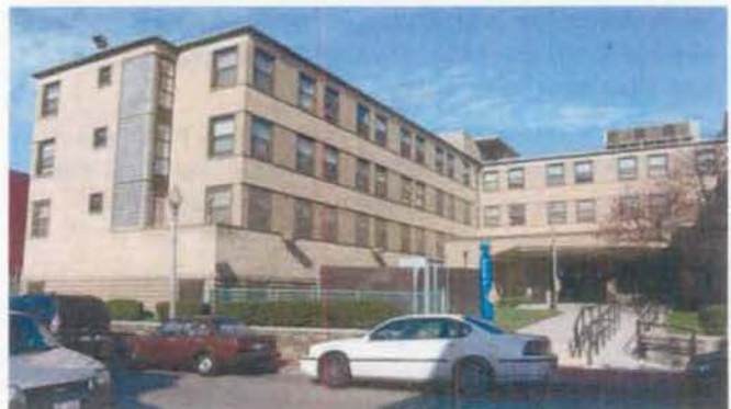
Photo 4-15: Carver Hall, 211 Elm Street. Built 1942 (History Matters, LLC, November 2009.)
