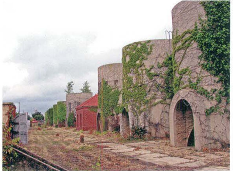
Photo 4-24: View of Sand Filtration Plant Silos at McMillan Reservoir
