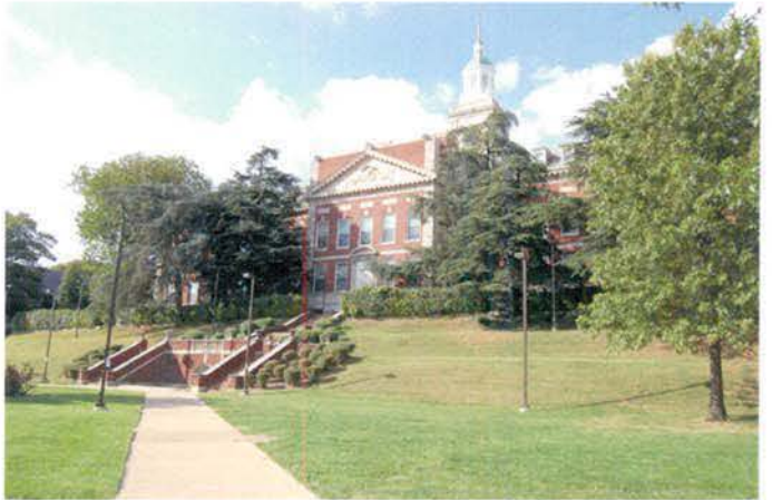
Photo 4-29: Founders Library, South elevation - overlooking Lower Quadrangle (History Matters, LLC, October 2009)
