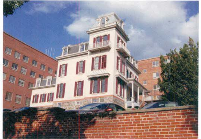
Photo 4-28: Howard Hall looking northeast from Georgia Avenue (History Matters, LLC, October 2009).
