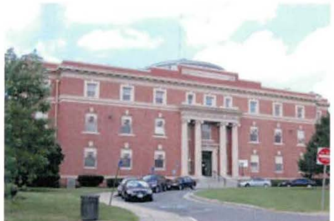
Photo 4-26: Former Freedman's Hospital, south elevation of central block (History Matters, LLC, October 2009).
